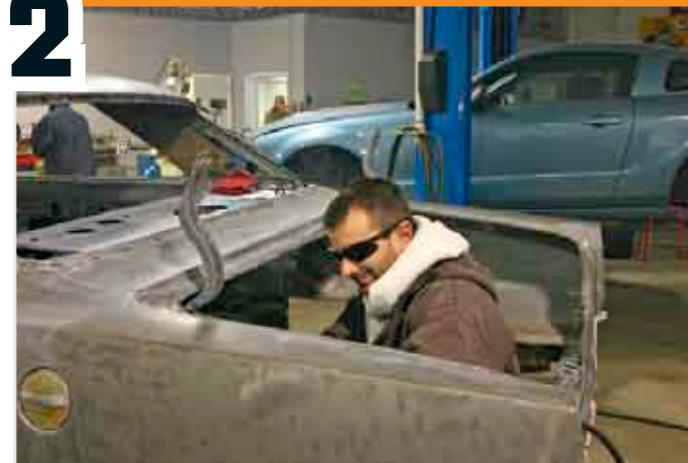
At first we thought Ed wanted to see how many bodies could be fit into the trunk, but believe it or not, he was getting down and dirty cutting out the trunk pan. The rear framersails were also removed at this time to make room for the new "real" frame section.
